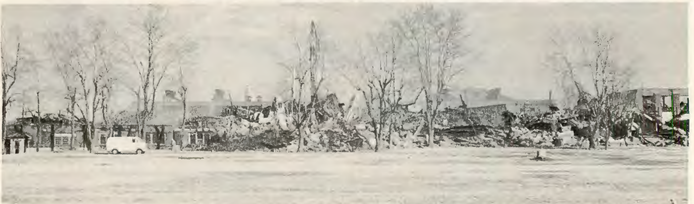
Eleven seconds after detonation, Donovan has created a mound of broken brick, twisted steel, splintered wood and shattered glass.
